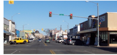
4th & Lewis – Downtown’s 100% retail corner. Northside anchor is the Franklin County Courthouse.
