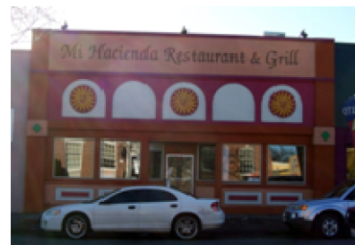
Great example of a nicely completed facade – ready for occupancy by a new business tenant.
